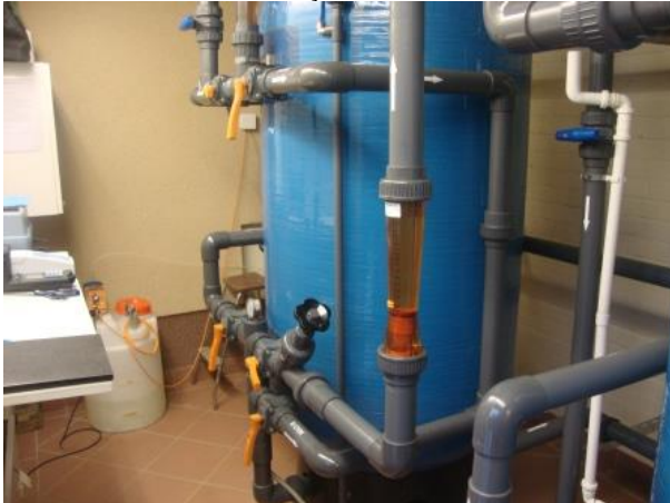
Water filters in the auxiliary structure
